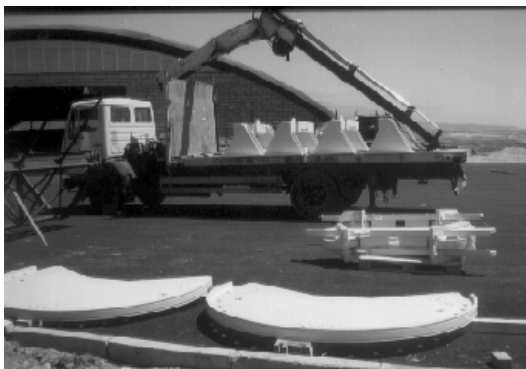
Figure 7: Carrying the first driving mechanisms form ITER workshop to the field.
